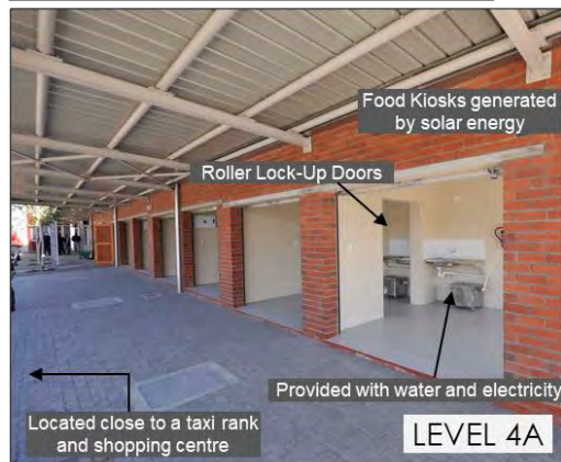
Cape Town - Nomzamo Business Area
