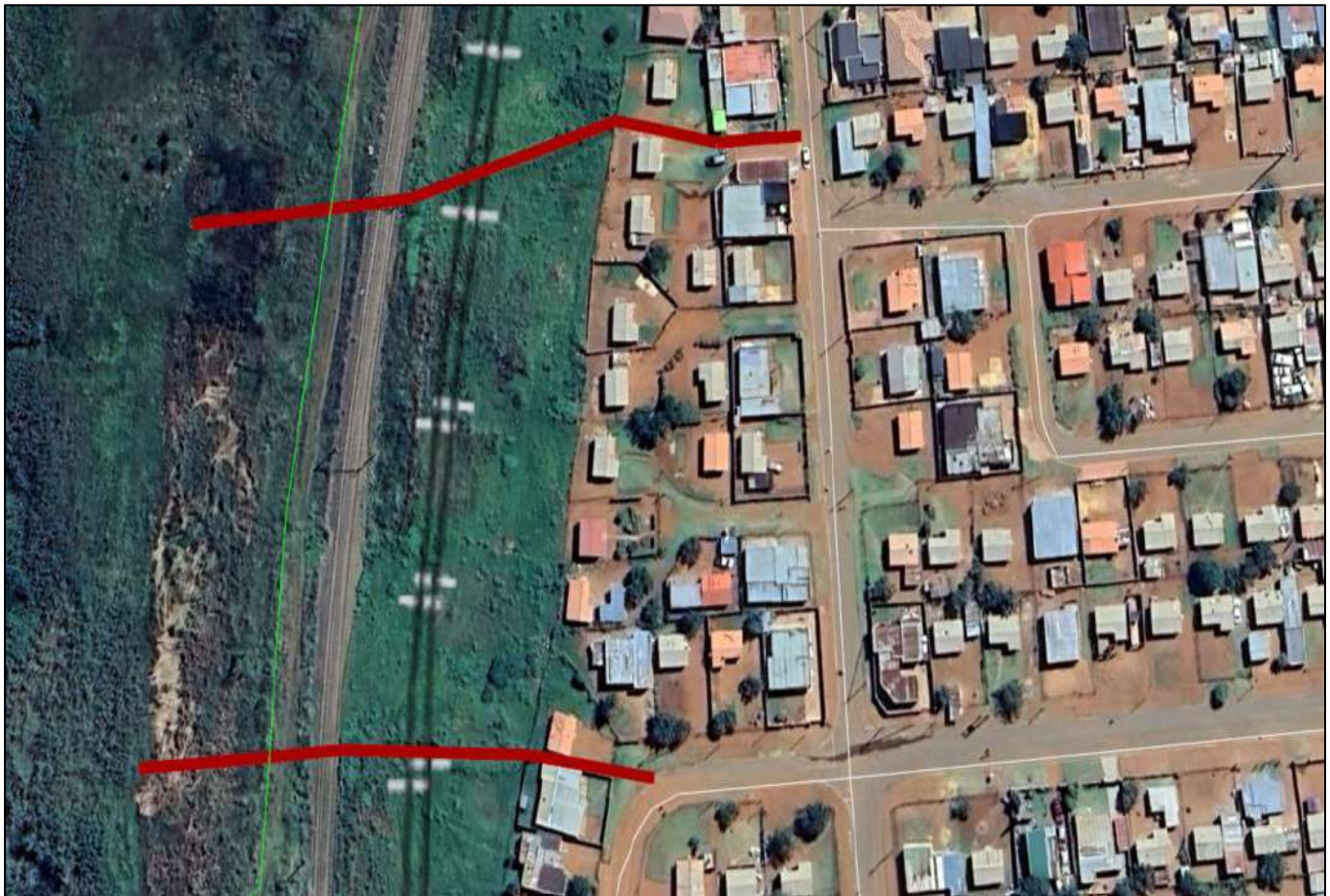
Priority 1: WARD 6 Lakeside Stormwater Open Channel/Culvert System
