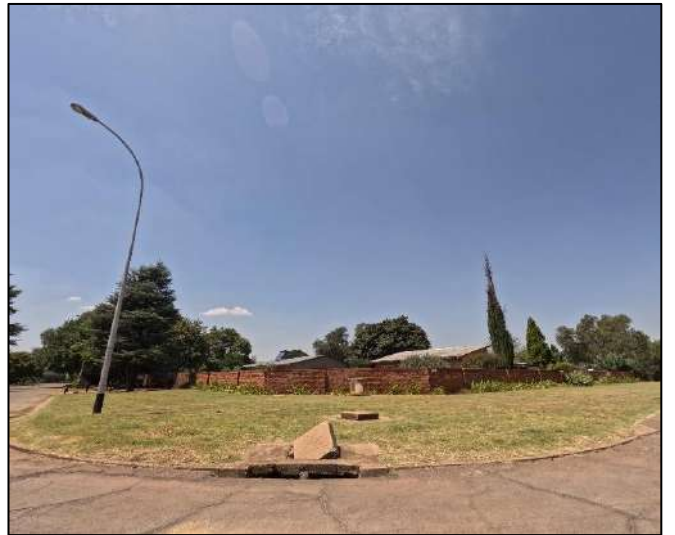
Figure 20: Stormwater Channels Blocked, Crocodile Cracks on Road Surface and Damaged Kerb Inlets
