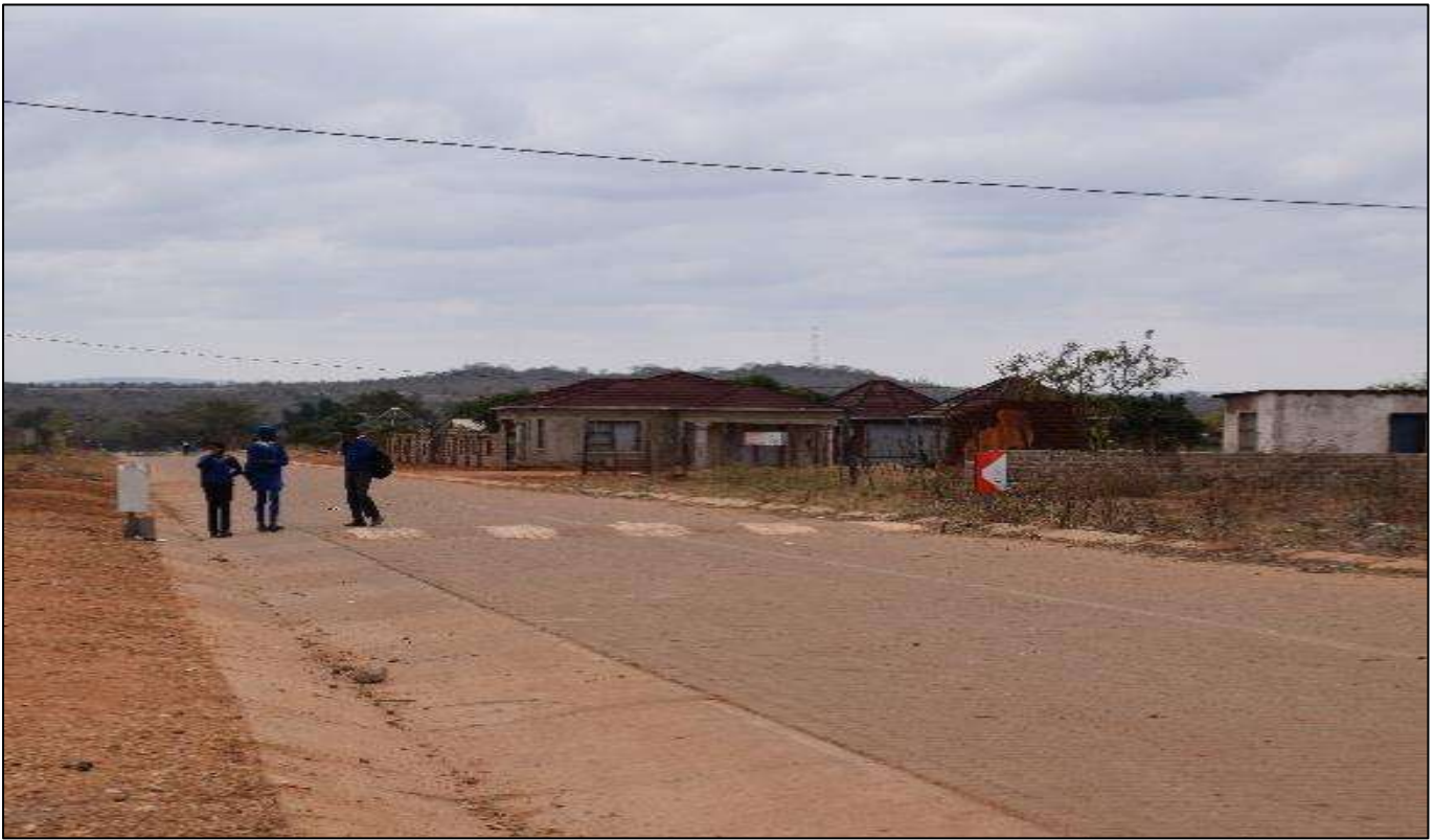
Figure 62: Example of a Concrete drainage channel implemented next to a surfaced road.
