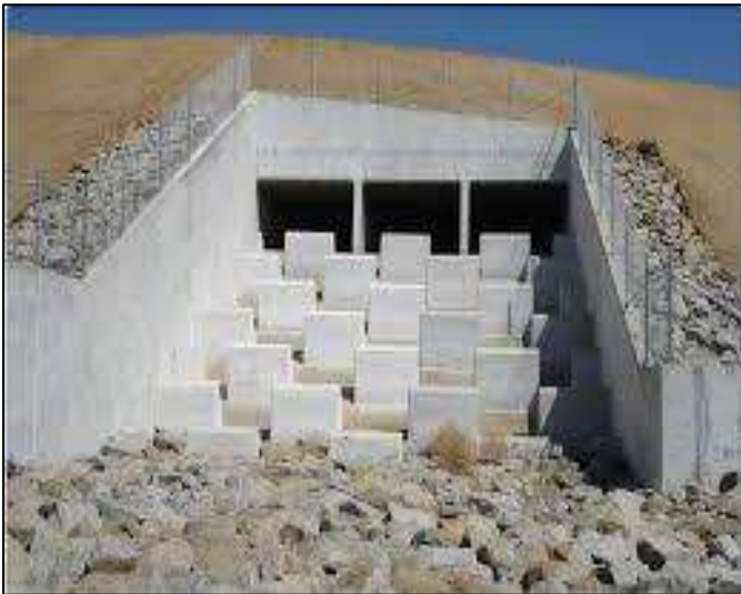
Figure 63: Typical Example of Energy Dissipation Structure
