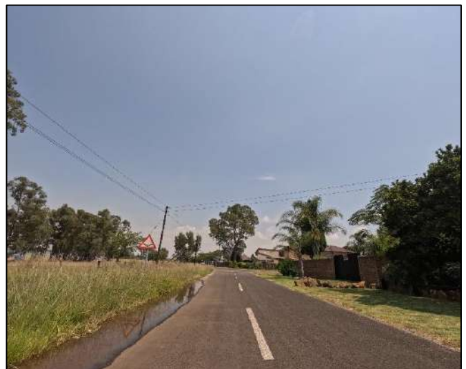
Figure 18: Stormwater Channel Damaged and Ponding on Road Surface
