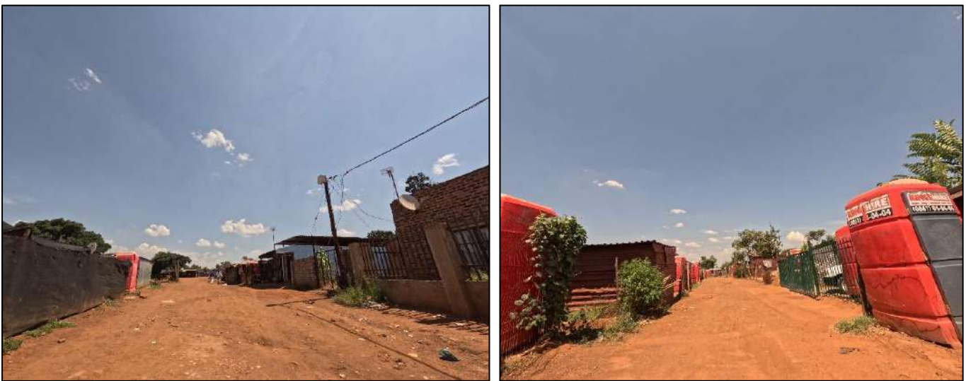
Figure 46: Roads Not Graded Properly and No Stormwater Drainage
