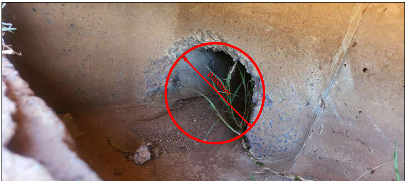
Figure 23: Stormwater Outlet Pipe to Small
