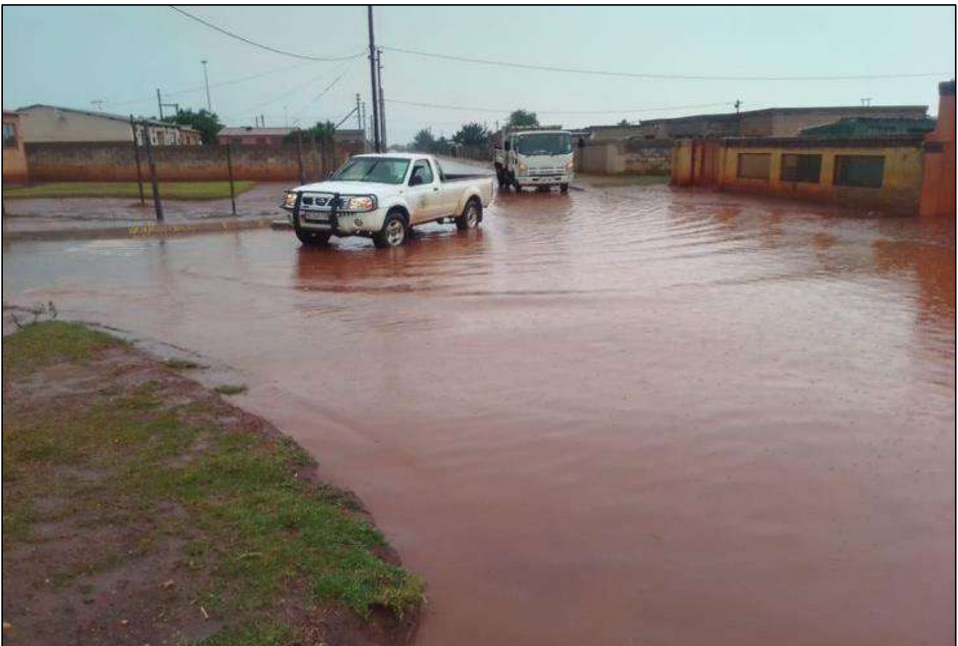
Figure 30: Overflowing Due to Insufficient Capacity
