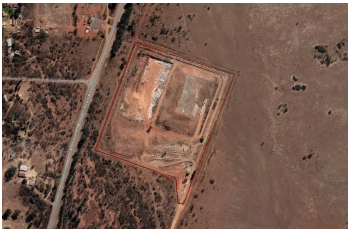
Figure 24: Walkerville landfill site (data source: Google Earth, accessed on 03/12/2005)
