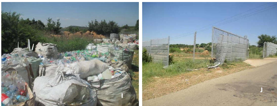
Figure 27: Photo A: Visual impact of site, B: clearing of waste on site, Photos C & D: recyclable material recovered by informal re-claimers on site, Photos E: quarry where cover material is mined from is also used as a wet weather cell. Photo G: powerline traversing the site. Photo H: water ponding noted in the wet weather cell. Photo I: TLB in use on site. Photo J: PET recycled from site. Photo K: damaged south western boundary of the fence.
