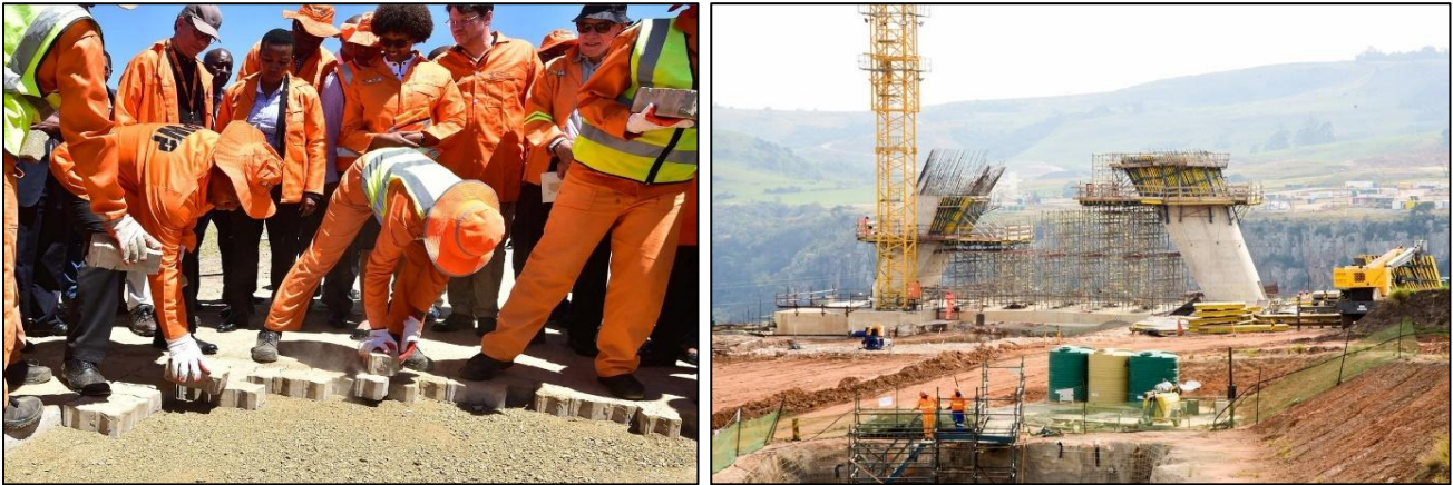
Figure 44: Public works infrastructure projects of a local road and N2 Msikaba bridge
