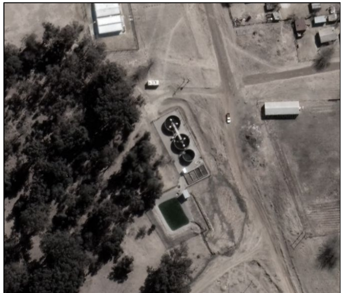
Figure 33: Waste water treatment plant in Bantu Bonke
