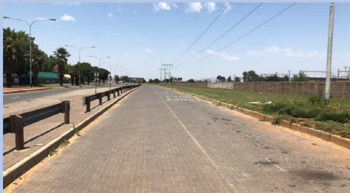
Lane for trucks next to station (also used by taxis)
