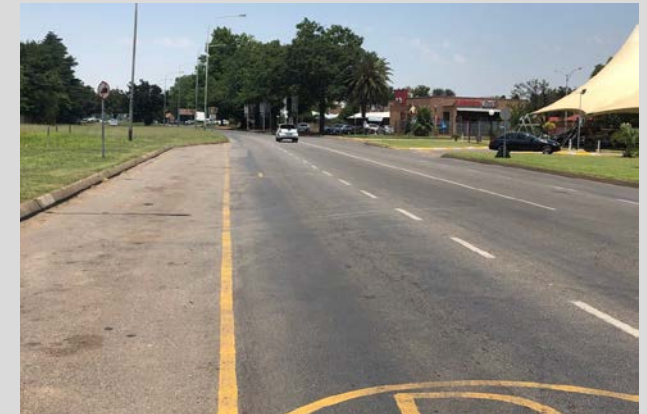
Extended bus/taxi lay-by next to Pierneef Boulevard with shelter
